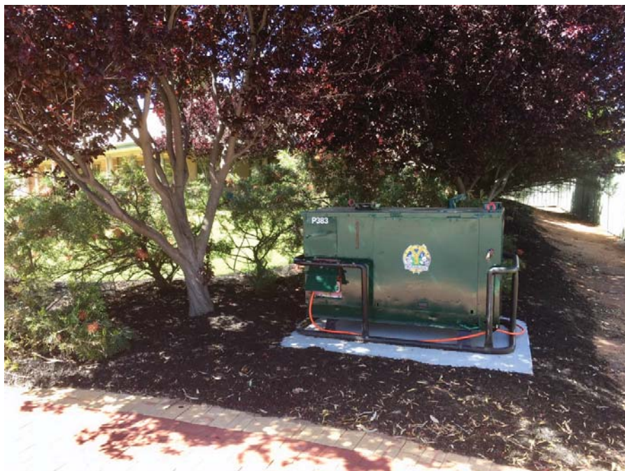
Generator – painted and on new concrete pad
